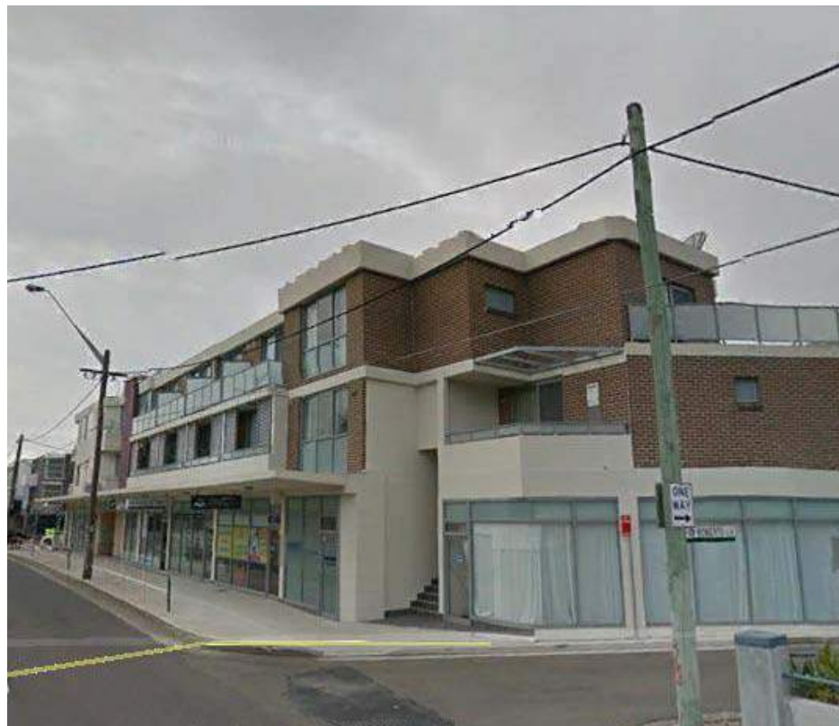
45-51 Forest Road (north of subject site) viewed from near intersection of Forest Road and Roberts Lane
