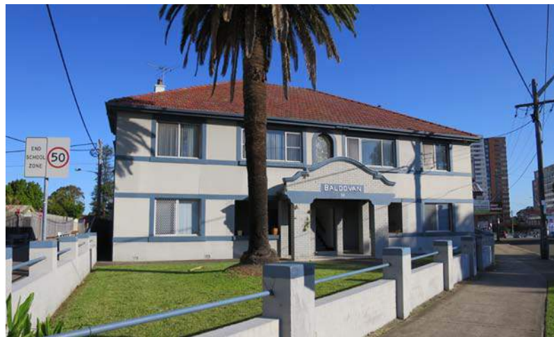
Existing residential building at northern corner of site
