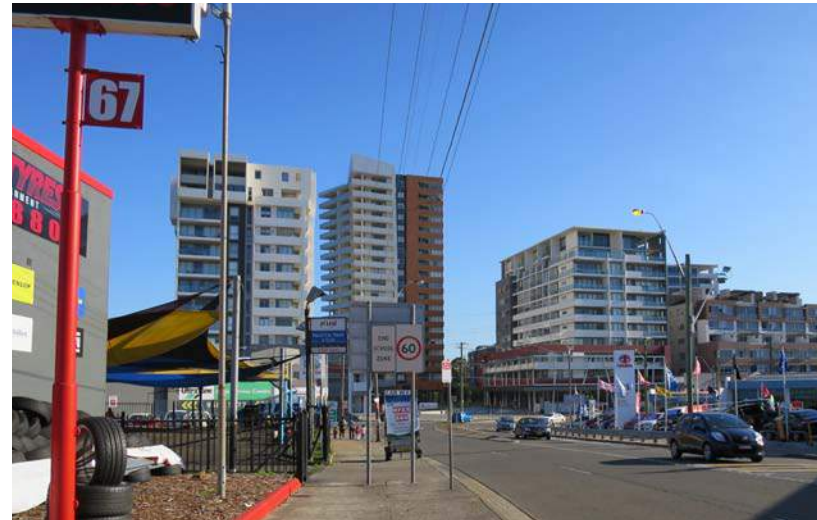
View looking south from footpath adjacent to subject site showing existing automotive uses fronting Forest Road
