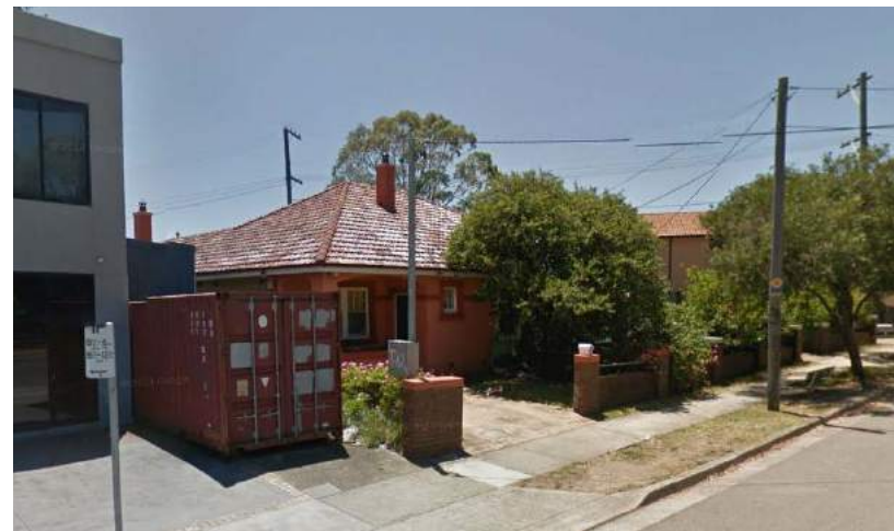
Existing residential building at eastern corner of site
